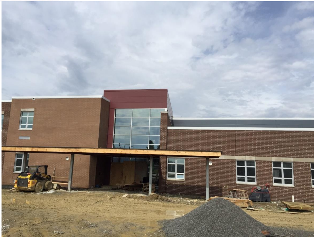
Roof coping and siding
