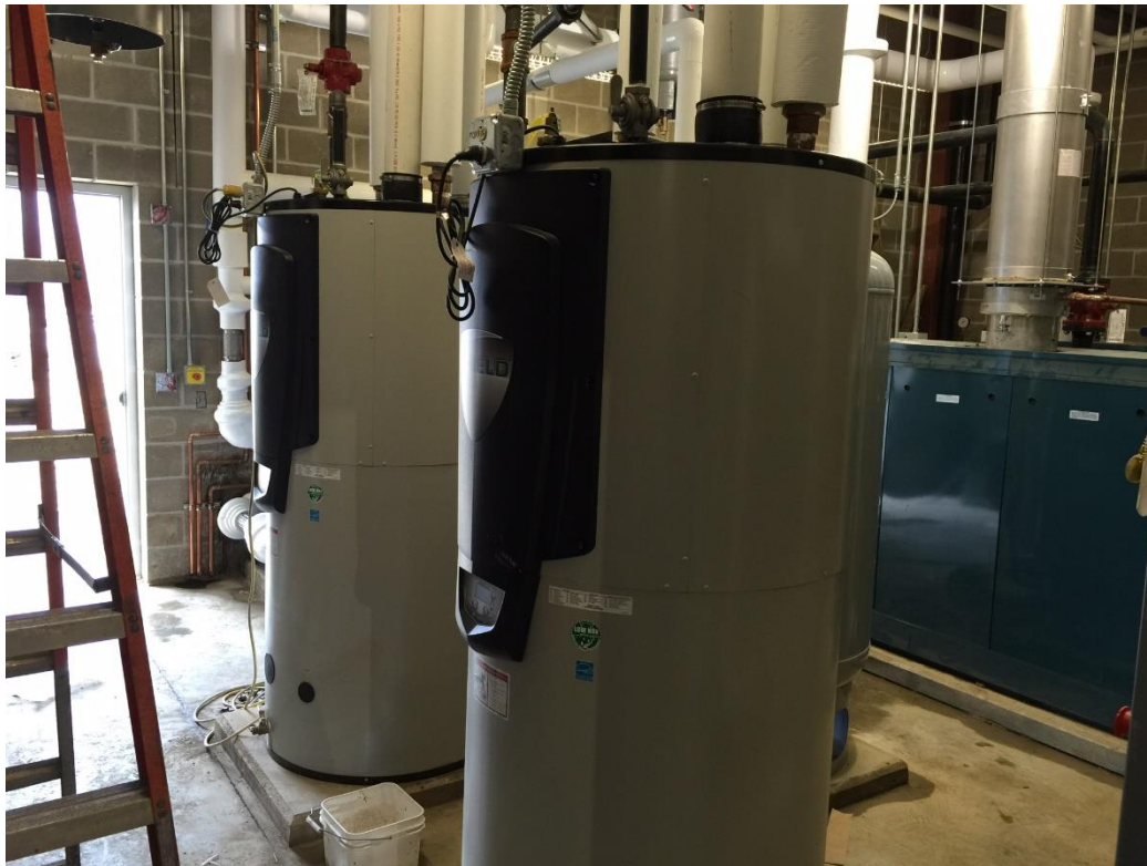
Hot water tanks and boilers
